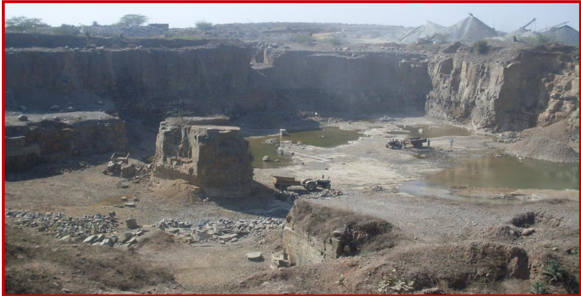
Fig. 3: Working Pit showing open cast mining activity
